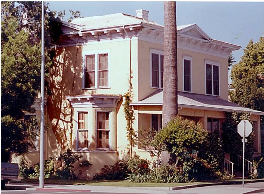
The Marysville residence of the family of Leonhard Scheu as it appeared in 1998. The location is 204 5 th St., at the southwest corner of 5 th and B.
